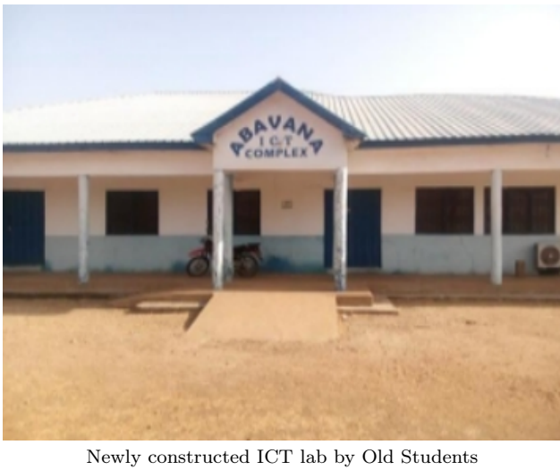
Figure 3. The ICT laboratory which was constructed by old students to aid in digital learning in the school. The laboratory houses a small number of computers and accessories.
