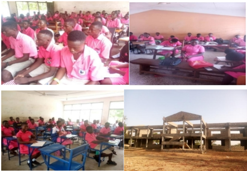
Figure 6. Students studying in an overcrowded class, others sitting on benches while others using tables and chairs provided by PTA, and a new classroom block under construction.
